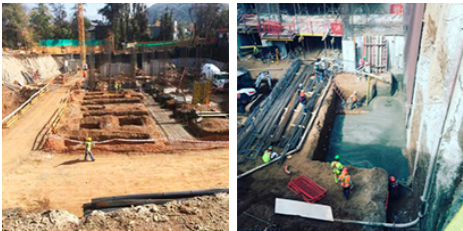
Placing and vibrating of concrete for foundations
