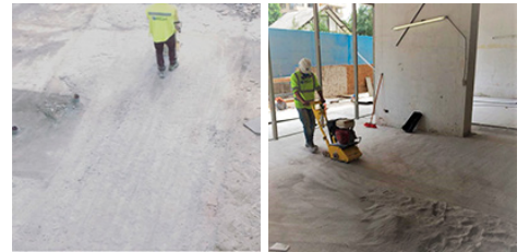
Scarification service and removal of paints and / or pre-existing membranes
