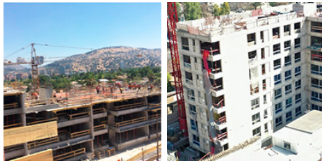
Concrete placement for high-rise edifications, full service
