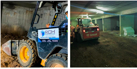
Preparation, levelling, and compacting of support (base and sub-base)
