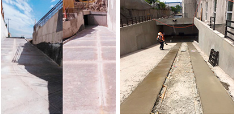
Ramp execution service
