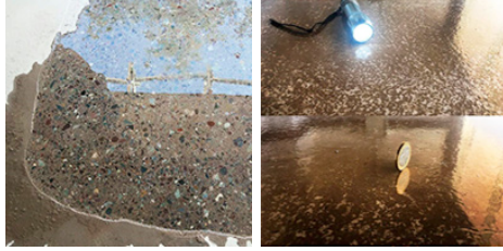
Dry polishing of concrete with different finishes
