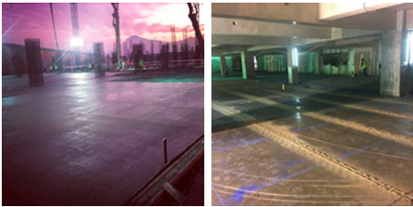
Concrete refining in slabs and foundations
