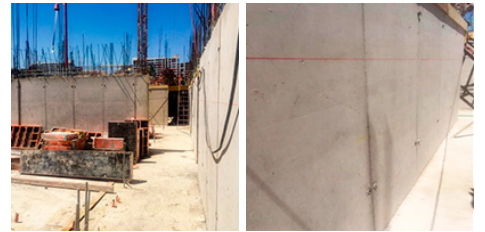
Placing and vibrating concrete in walls against ground and two faces
